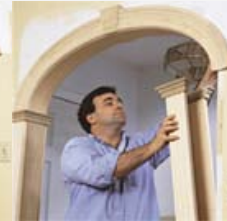
Slip arch columns under header.
