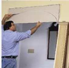
Remove columns; cut out sheetrock; patch.
