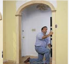
Level horizontally; nail all parts into place.
