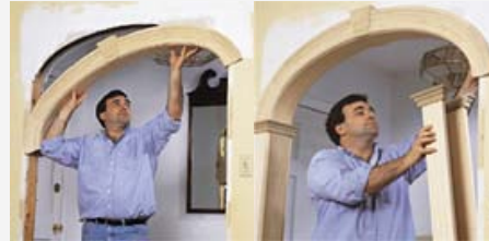
Slip arch header onto wall.
